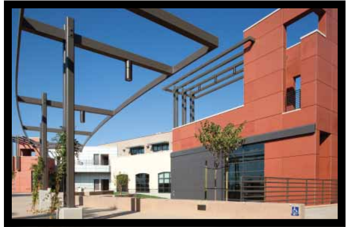
Miramar College Hourglass Park Field House
